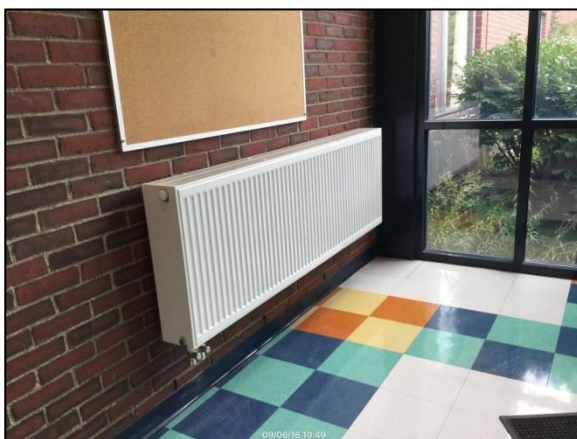
New radiators in South School
