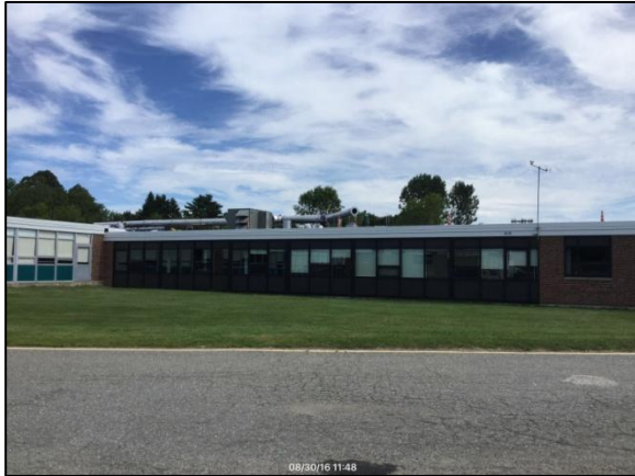
ERVs and ductwork on roof - OHS
