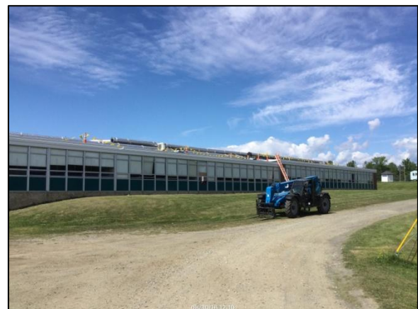
Ductwork being installed on the roof at OHS
