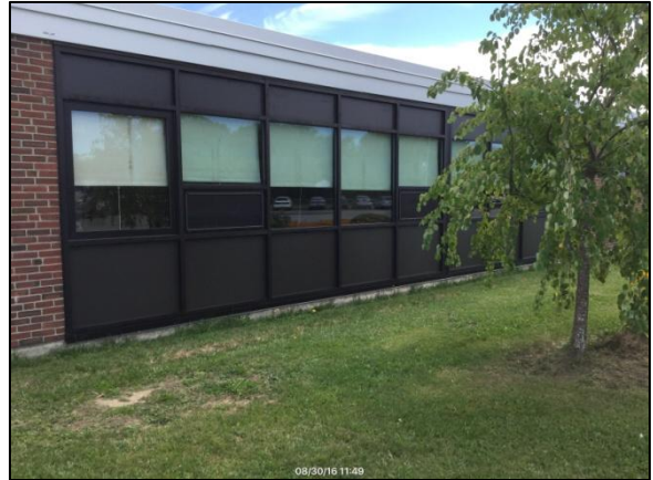
New windows at OHS
