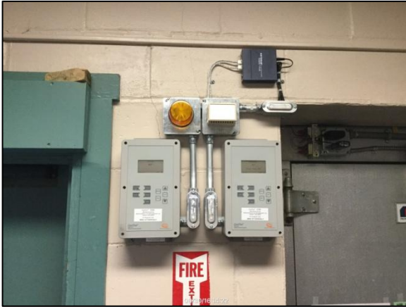
Refrigeration controls
