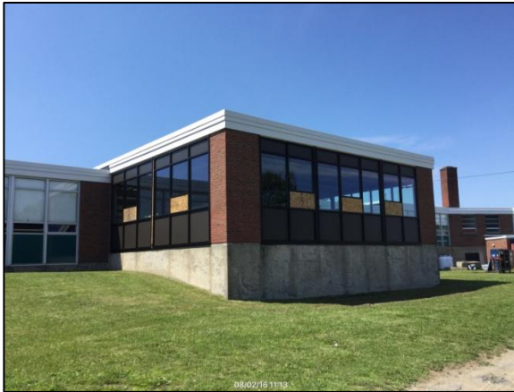
New windows installed in HS library
