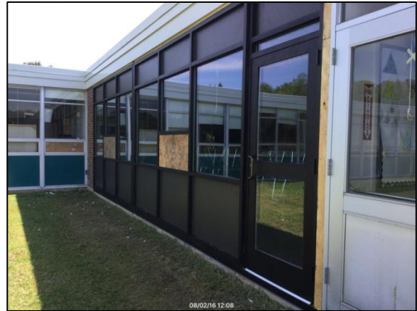
New windows installed in HS classroom 21
