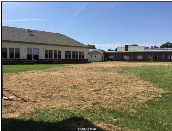
Ground surface replaced over underground piping
