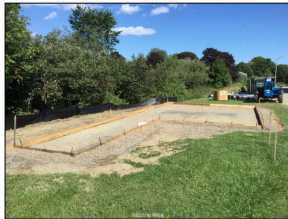
Pad prep for tank farm at OHS
