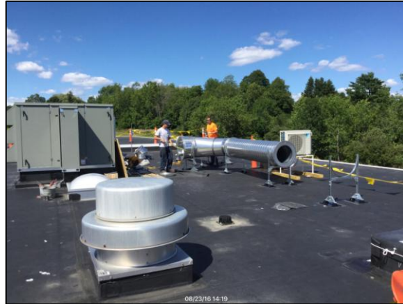
Roof-mounted ductwork installation at OHS
