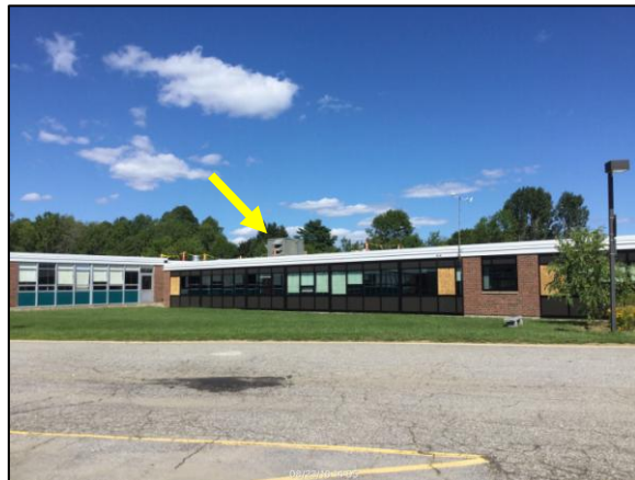
HVAC equipment on OHS roof
