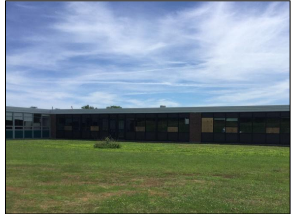
New windows at OHS - Rear elevation (operable portions to be installed)
