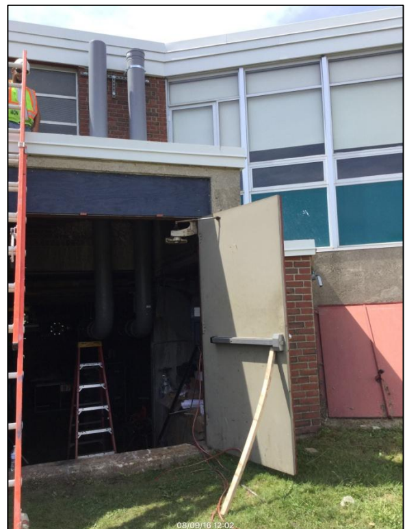
Installation of boiler room ventilation stacks at OHS
