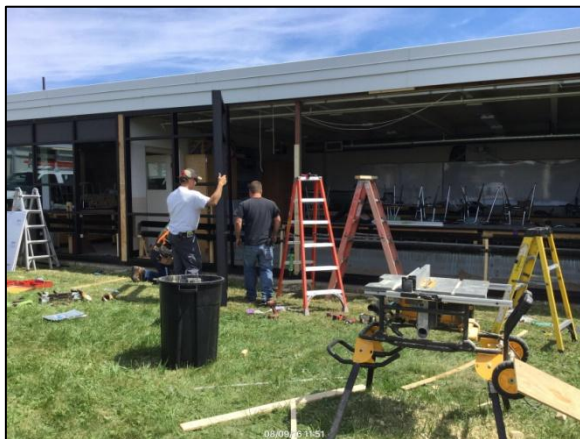
Installation of windows in front classrooms at OHS
