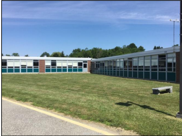
Old windows at OHS - Rear elevation
