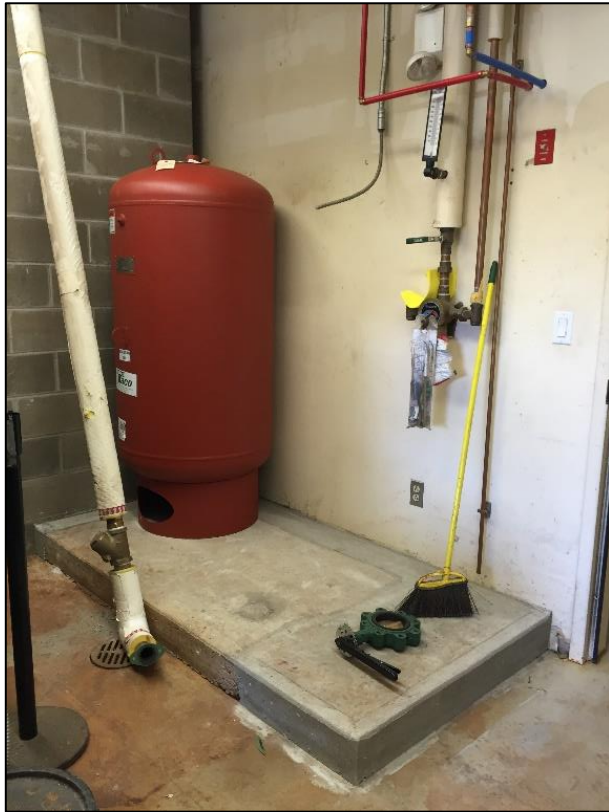
New extended slabs and water tank - South School boiler room
