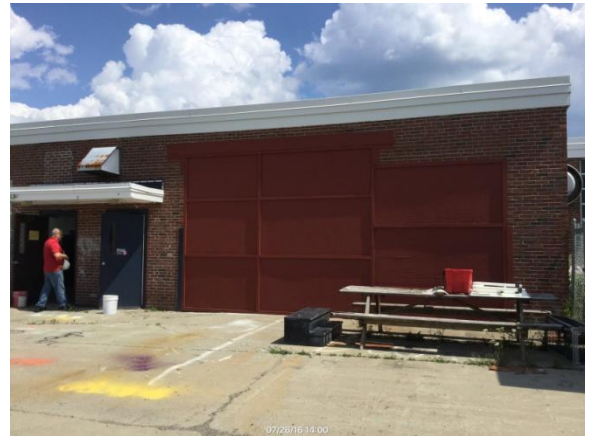
Removal of overhead door and construction of exterior wall at Oceanside Middle School
