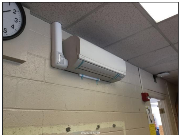
Ductless splits are being installed
