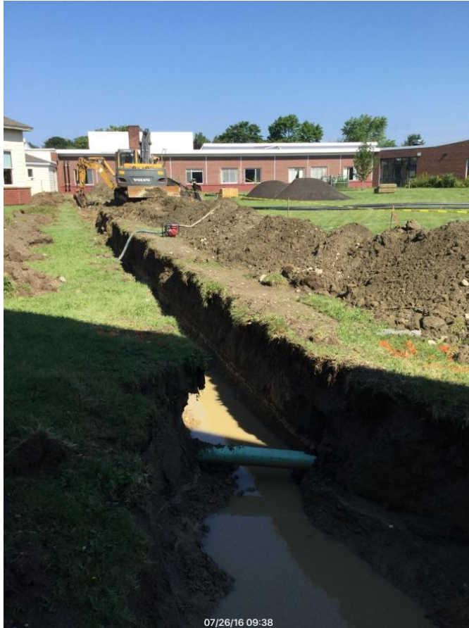
Installation of underground piping at South Elementary School
