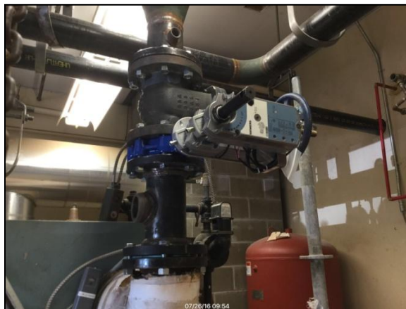
New automated isolation valves are installed
