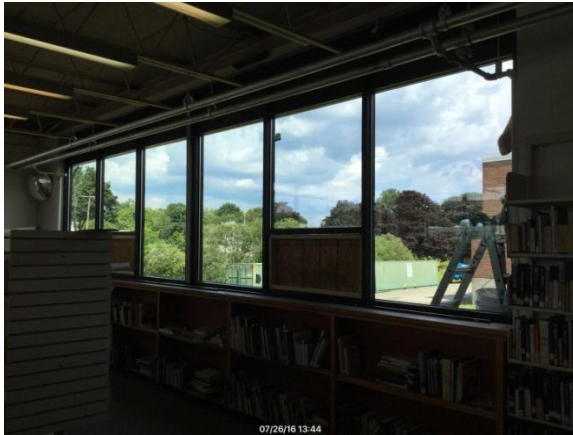
New windows being installed at the high school
