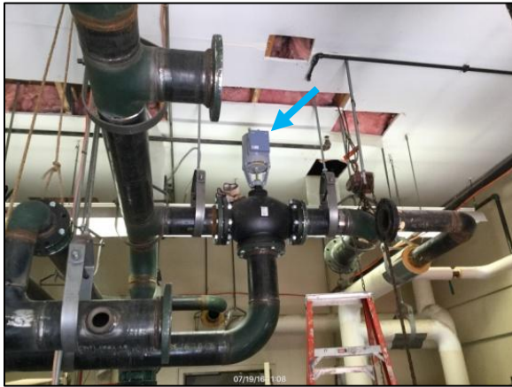
3-way valves installed in the boiler rooms
