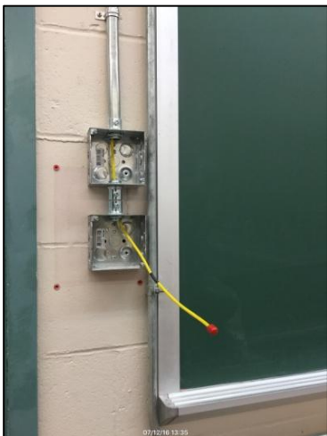
Wiring and installation of controls is ongoing throughout the schools
