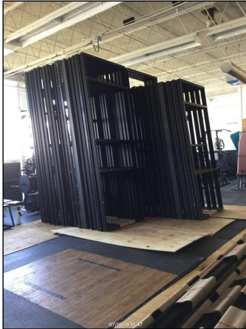
New window frames on site at Oceanside High School
