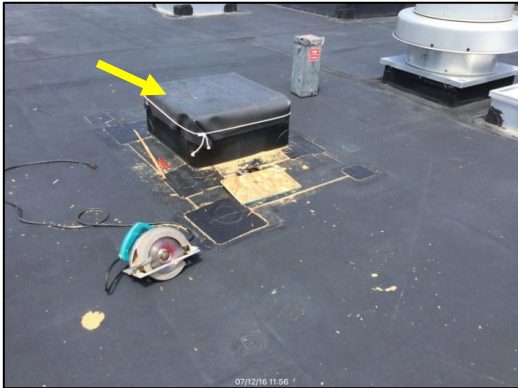
Roof penetration for ventilation - exterior
