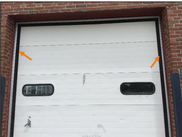
Weatherization of overhead door at OHS East
