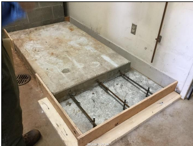
Pouring new slab for tanks in middle school boiler room
