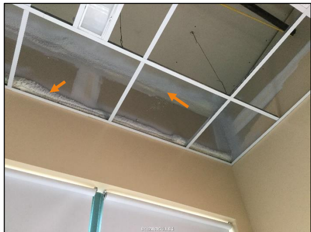
Foam sealing in cafeteria at RDMS/South School
