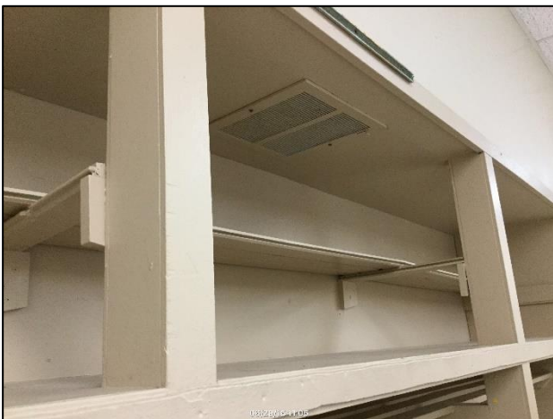
Sealed above classroom vents in RDMS
