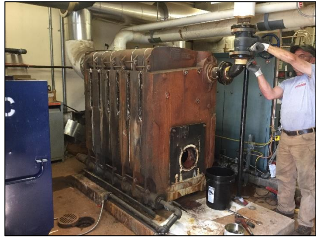
Removal of oil boiler - RMS
