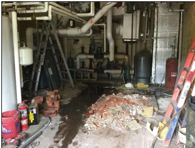
Removal of oil boiler - TGS
