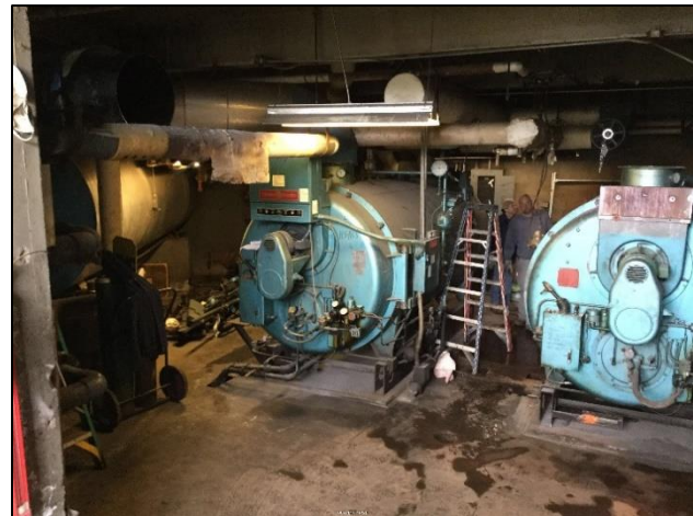
Removal of oil boiler - OHS East
